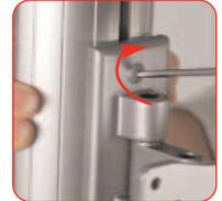
Once in position, tighten the bracket onto the linear post
